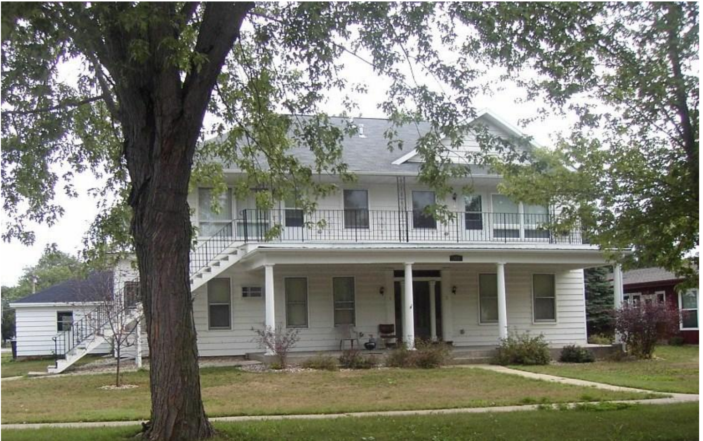
The D.G. James House as a four unit apartment Building – SandHill Marketing
