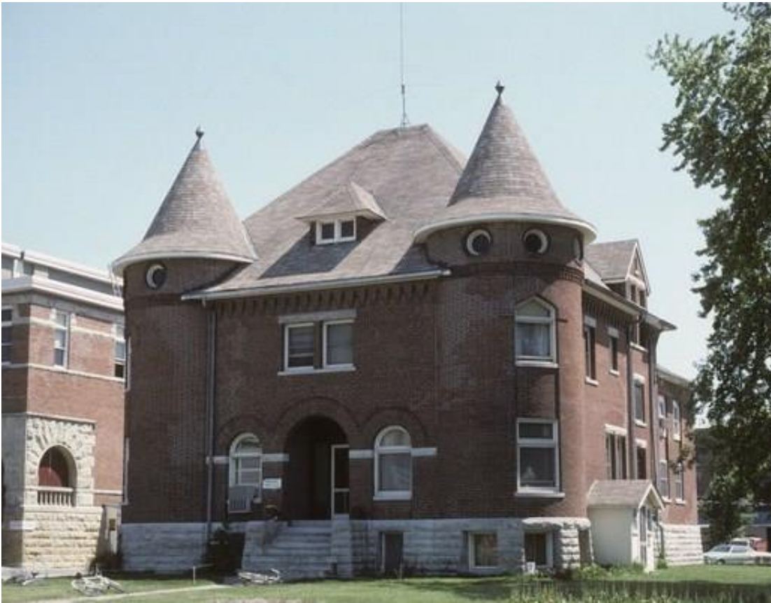
Richland County Sheriff's Office and Jail, 179 West Seminary Street, 1904, 1981. Designed by Andrew Lew Porter in the Romanesque Revival style, this red brick hip roofed rectangular building is characterized by twin round two-story towers with conical roofs, small round frieze windows and Tudor arched windows that flank the facade. Corbeled brick white stone lentils and sills, a white stone elevated foundation, and a triple arched entrance further characterize this well
