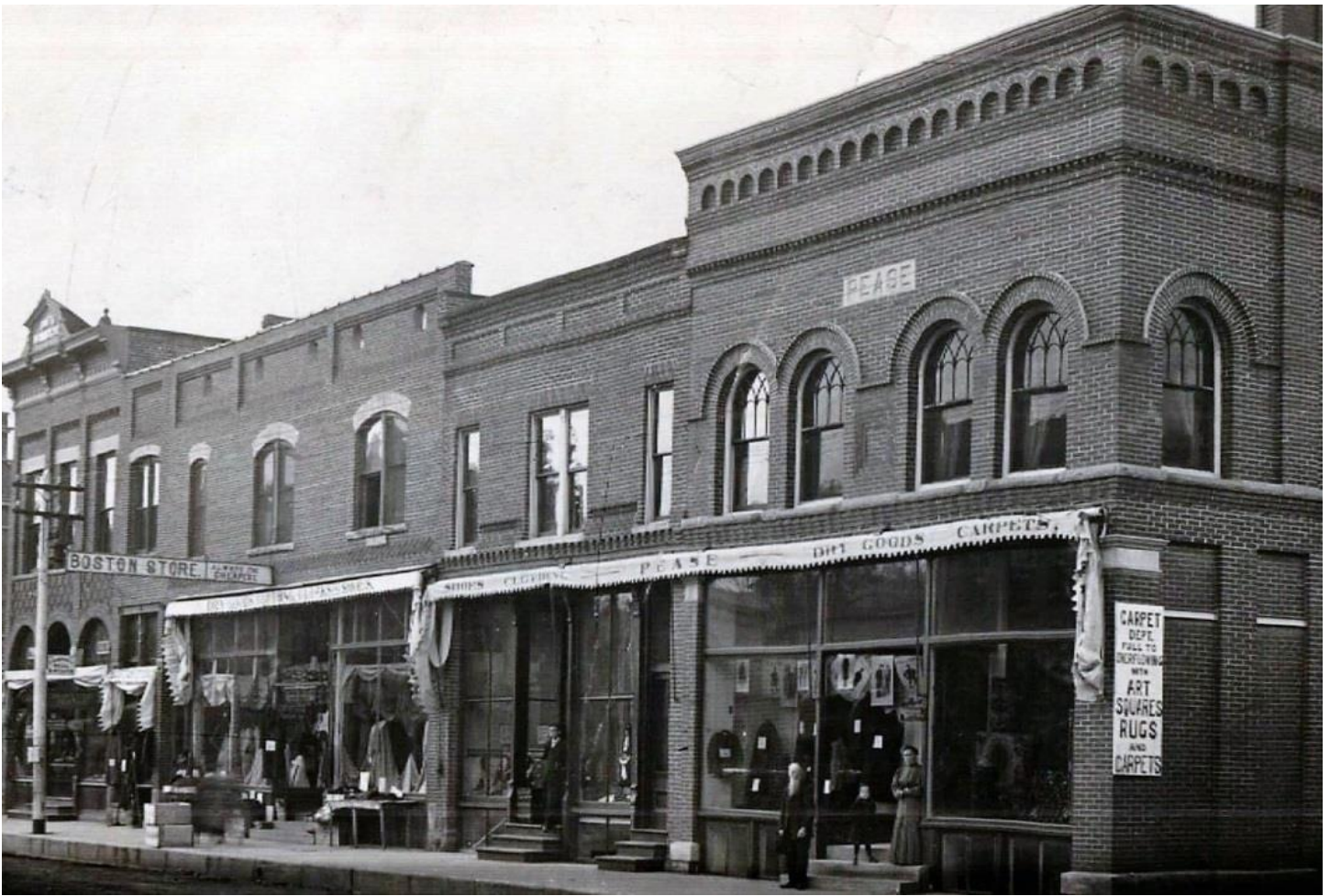
D.E. Pease Store, 172 West Court Street, 1899. Featuring Romanesque Revival influenced round arched windows with brick voussoirs and moldings, this brick two-story building is further characterized by a wide projecting brick cornice ornamented by a blind arcade as well as ornamental brick work. Although historically significant, this building is not architecturally significant because of the extensive alteration of the storefront and the removal of the arcaded parapet and leaded windows. Historically significant for its association with the Pease store originally established on the site in the 1850s, the building continues to serve as a general merchandise store.
