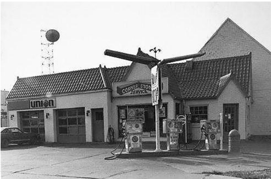
LeHew Filling Station, 208 South Church Street, 1927. Characterized by a red tile roof and multiple gables, this (originally) white brick Tudor Revival/Mediterranean styled gas station has examples original multi-paned windows remaining on the building. The large service door and main storefront window have been replaced. The LeHew Filling Station was constructed by Dell Beaty in 1927. The building has been remodeled a number of times, removing much of its original architectural detail.
