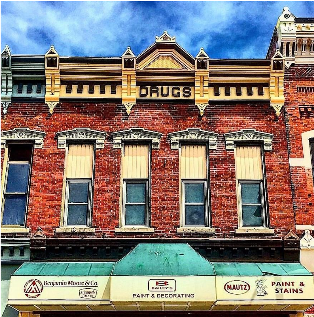
Burnham and Burnham Drug Store, 182 East Court Street, 1889, 1892. Ornamented by a large projecting metal cornice characterized by a triangular pediment and bracket trim, this two-story Italianate styled brick building is further ornamented by triangular pediment shaped window heads and a small cornice extending across the storefront. An addition located at the rear was constructed in 1892. Iron columns flank the entrance of the otherwise completely remodeled storefront. Although the architectural character of the building has been compromised by the second story replacement windows, this building used as a drugstore until 1962, continues to exhibit a strong Italianate character.
