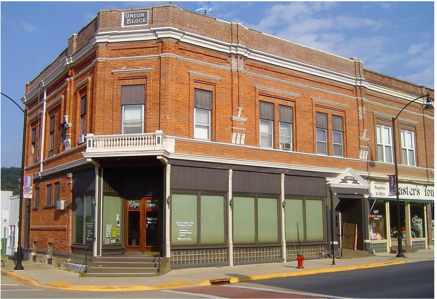
Union Block, 100-124 North Main Street, 1892, 1911. Exhibiting a rather eclectic manner, this two-story Classical Revival influenced vernacular brick block features a plain projecting brick cornice and parapet resting on applied brick pilasters, which vertically divide the brick surfaces of the upper story. Window cornices, raised brick moldings, a wooden balcony over the corner entrance and a frontispiece in a classical design further characterize the building. Capped brick pilasters and cast iron columns remain on the storefront. An addition built in a style similar to the original building was constructed on the north end in 1911. Built as rental property for W.H. Pier and Laura McCarthy, the Union Block has housed several long-term businesses.
