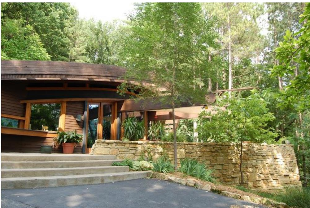
The house has curved walls and a curved roof matched with curved exterior beams laminated at the job site. It faces south and the large expanse of glass helps keep the living space comfortably warm. The home is fitted with a radiant heat system built into the tile floor.
